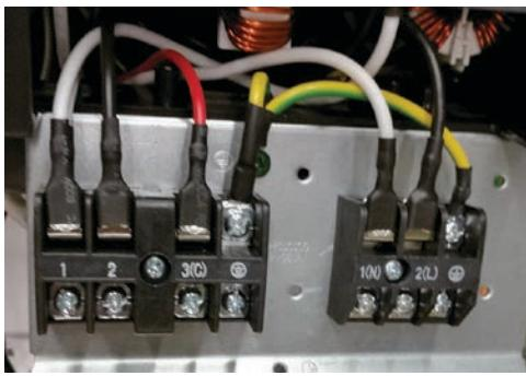
The outdoor unit is powered by 208/230 Volt Single Phase electricity connected at the Outdoor Unit Terminal Block. Terminals 1 and 2 on the outdoor unit terminal connect this voltage to the system. The number 3 terminal is a communication terminal that connects wiring between the indoor and outdoor units. An earth ground source terminal connects the outdoor unit to the line voltage power source.
