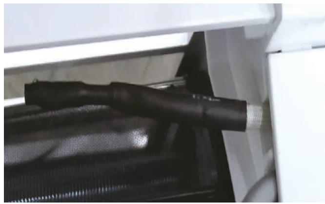
The Room Ambient Temperature Sensor is a negative coefficient thermistor that will decrease in resistance with increases in room air temperature. The sensor is located on a clip mounted to the surface of the indoor coil.
