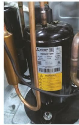
The compressor is a three phase DC inverter driven Rotary type. The compressor is capable of variable speed operation. The compressor operating frequency will be determined by the temperature difference between set point and room or outdoor air temperature. (Cool Mode versus Heat Mode)
