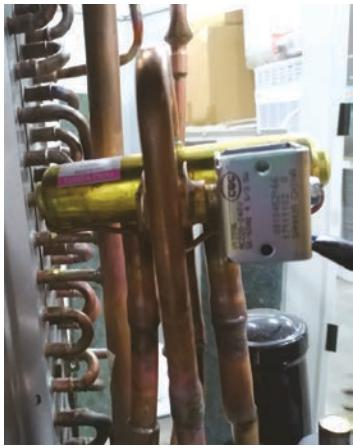
The 4-Way Valve redirects the flow of refrigerant in the piping circuit to allow the system to swap the functions of the indoor and outdoor coils. When de-energized in COOL MODE, the valve will direct the refrigerant hot gas to the outdoor coil. When energized in HEAT MODE, the valve will direct the hot gas to the indoor coil.
