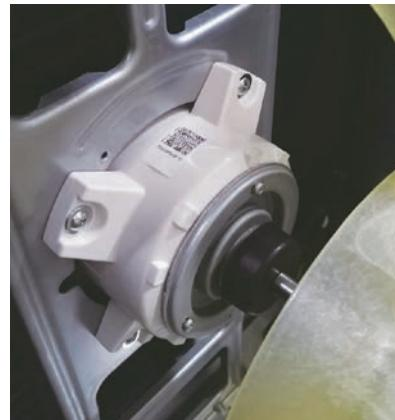
The outdoor fan motor is a variable speed motor. The required motor speed is calculated by the Main Control Board. The motor is electrically connected to the Main Control Board via PLUG CN-21.
