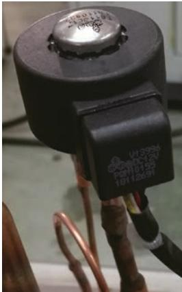
The metering device is an electronic expansion valve type EEV. The valve consists of an electrical operator and a valve body with internal variable size orifice. When operating, the Main Control Board will send pulses of voltage to the electrical operator. The operator will then magnetically move the position of the metering orifice pin to vary its size.
