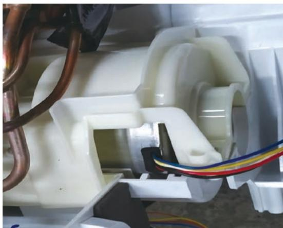
The Indoor Fan Motor is a variable speed motor. The motor will vary speed with the speed of the compressor inverter. The speed can also be set at the remote control or automatically adjusted using the AUTO fan mode. When in AUTO fan mode, the speed of the fan is calculated using the indoor set temperature and the indoor room ambient temperature. (Outdoor air temperature in heat mode.)
