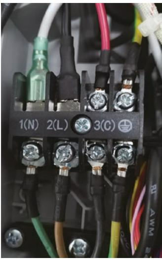
The indoor unit terminal block receives electrical power from the outdoor unit. There are 4 connections for electrical wires. Terminals 1 and 2 are connected to terminals 1 and 2 of the outdoor unit. This wiring supplies power to the indoor unit.
