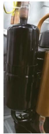
The Accumulator is located in the suction line circuit at the entrance to the compressor. The accumulator helps prevent liquid refrigerant from entering the compressor during run operation.
